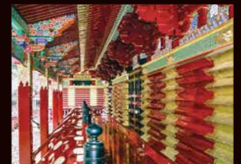
Toshogu Middle Sacred Storehouse After conservation repair work (2006)
