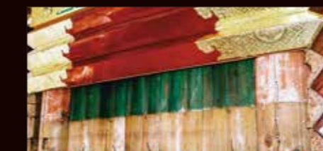
Middle Sacred Storehouse of Toshogu Shrine: The bay structure and painting remaining on the back side of the current logs used for this storehouse are proof of origin in the Edo Period, constructed by Lord Hidetada. These facts were discovered by a survey during repair work.
